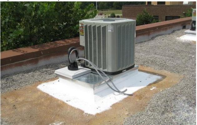
**Description:** The RTU (Roof Top Unit) is designed to supply a building with heat and air conditioning. The average life span of an RTU is roughly 15 to 20 years. The RTU's on top of the Astor Avenue Community Center have reached the end of their lifespan and are in need of being replaced. These RTU's are targeted to be replaced in FY 2019.
