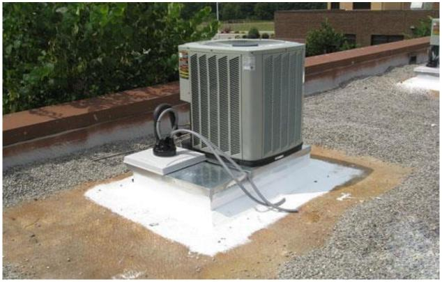
**Description:** The RTU (Roof Top Unit) is designed to supply a building with heat and air conditioning. The average life span of an RTU is roughly 15 to 20 years. A plan has been implemented to replace one RTU every two years, until all the old units have been replaced.
