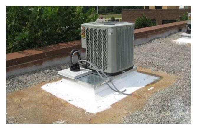
**Description:** The RTU (Roof Top Unit) is designed to supply a building with heat and air conditioning. The average life span of an RTU is roughly 15 to 20 years. A plan has been implemented to replace one RTU every two years, until all the old units have been replaced.
