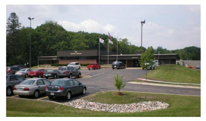
**Description:** The existing parking lot serving the Town Hall is in significant disrepair. Considerable reconstruction is required, including new asphalt paving, sealing, striping, and curb repair. In FY 2013, the lot around the Highway garages was reconstructed, and in FY 2016, the parking lot in front of the Town Hall is scheduled for reconstruction.
