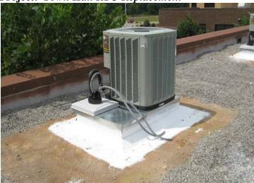
**Description:** The RTU (Roof Top Unit) is designed to supply a building with heat and air conditioning. The average life span of an RTU is roughly 15 to 20 years. In 2013 the Town Hall RTU will meet that age standard and at that time a determination will be made if and when a replacement is necessary.
