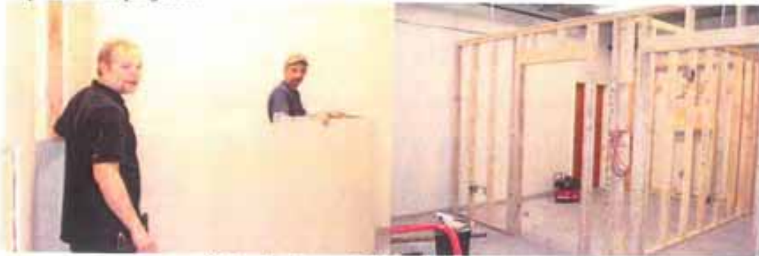
Pictured: Nurses Office Under Construction
