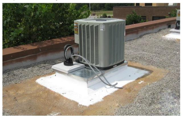
**Description:** The RTU (Roof Top Unit) is designed to supply a building with heat and air conditioning. Hanover Township's Town Hall building operates with 5 separate RTU's. The average life span of an RTU is roughly 15 to 20 years. A plan has been implemented to replace one RTU every two years, until all the old units have been replaced.
